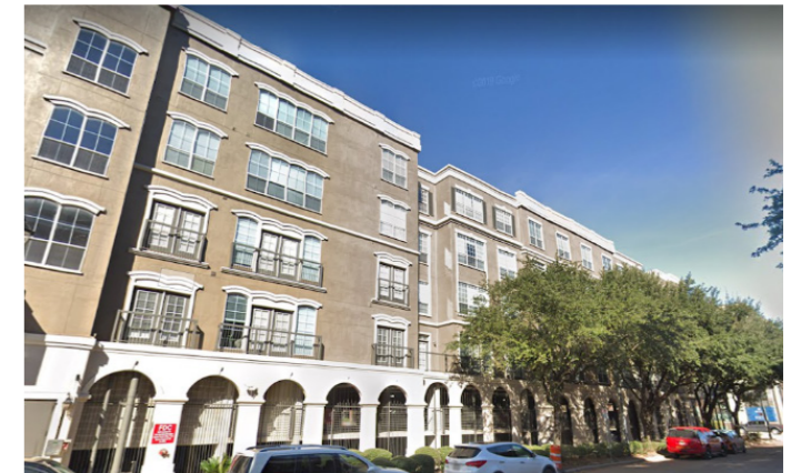
Fig. 3.9 | Louisiana St: New building typology introduced in Midtown
