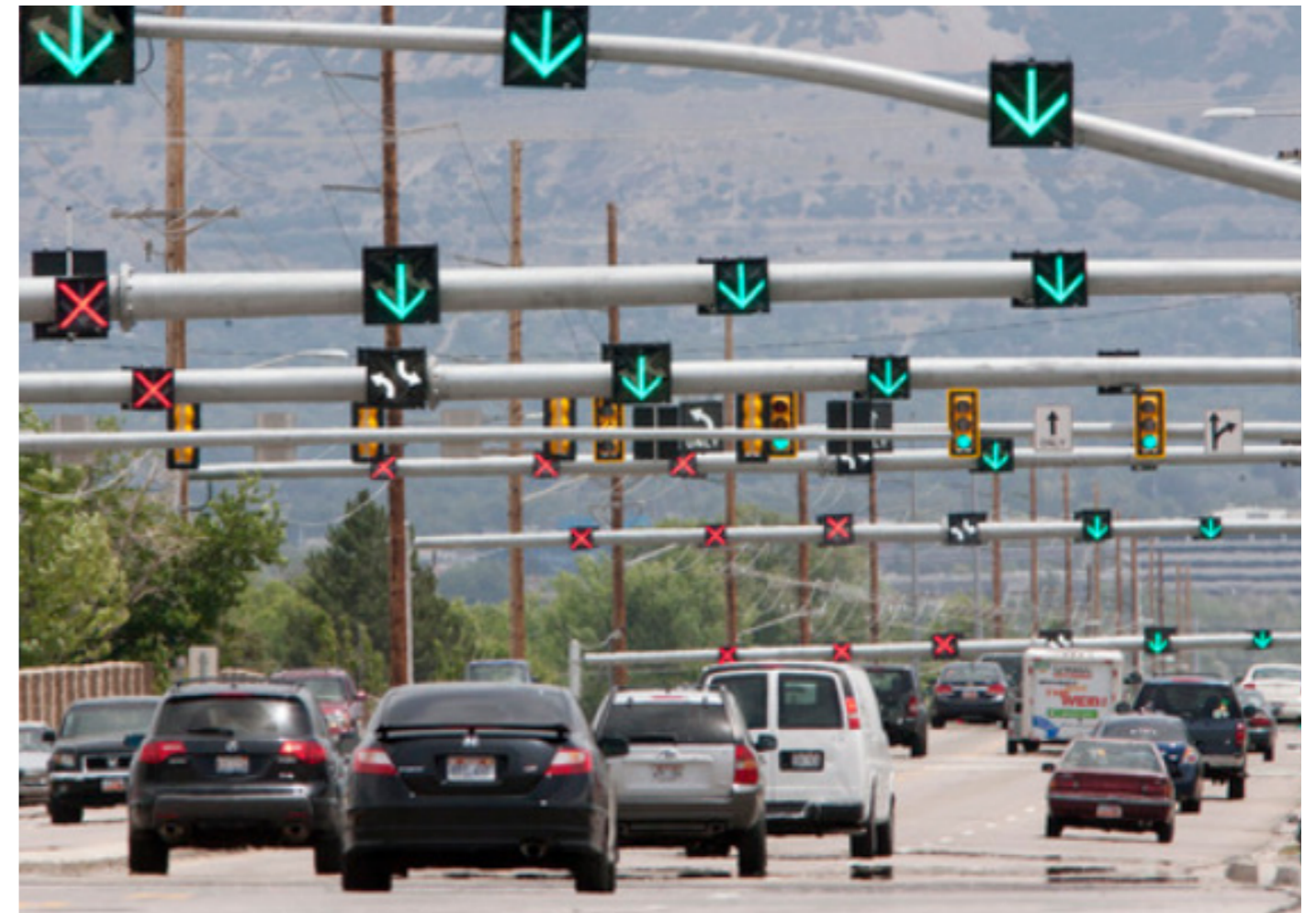
Fig. 4.24 | Reversible lanes system in practice in Taylorsville, Utah (Griffin, n.d.)
