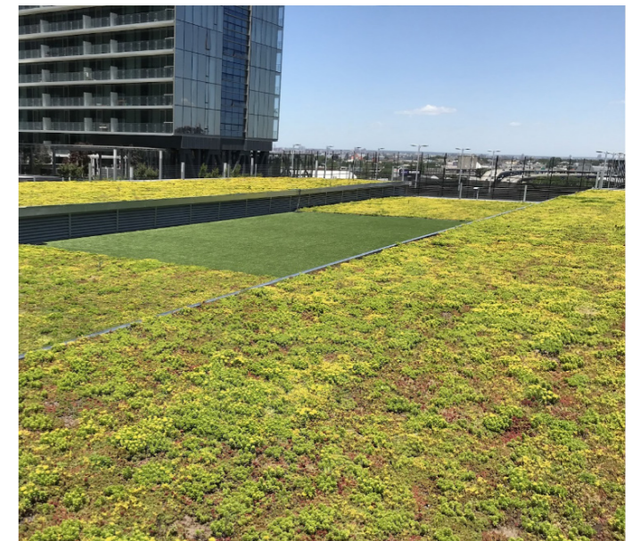
Fig. 4.38 | Green roof on top of a parking garage (Sempergreen, n.d.)
