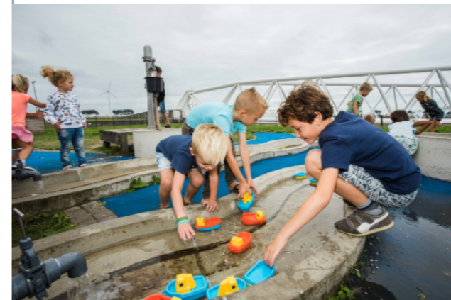
Fig. 4.3 | Water education park at Maeslantkering in Hook of Holland, the Netherlands (Het Keringhuis, n.d.).
