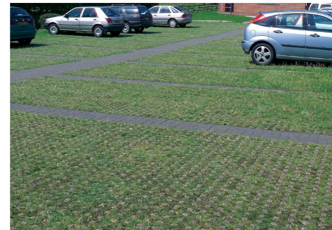
Fig. 4.39 | Semi-permeable parking lots (Green solutions, 2017)
