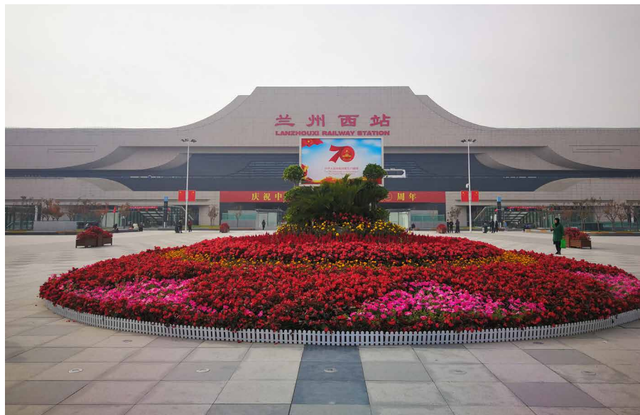
FIG. 5.3 Lanzhou West HSR station (Source: the authors)
