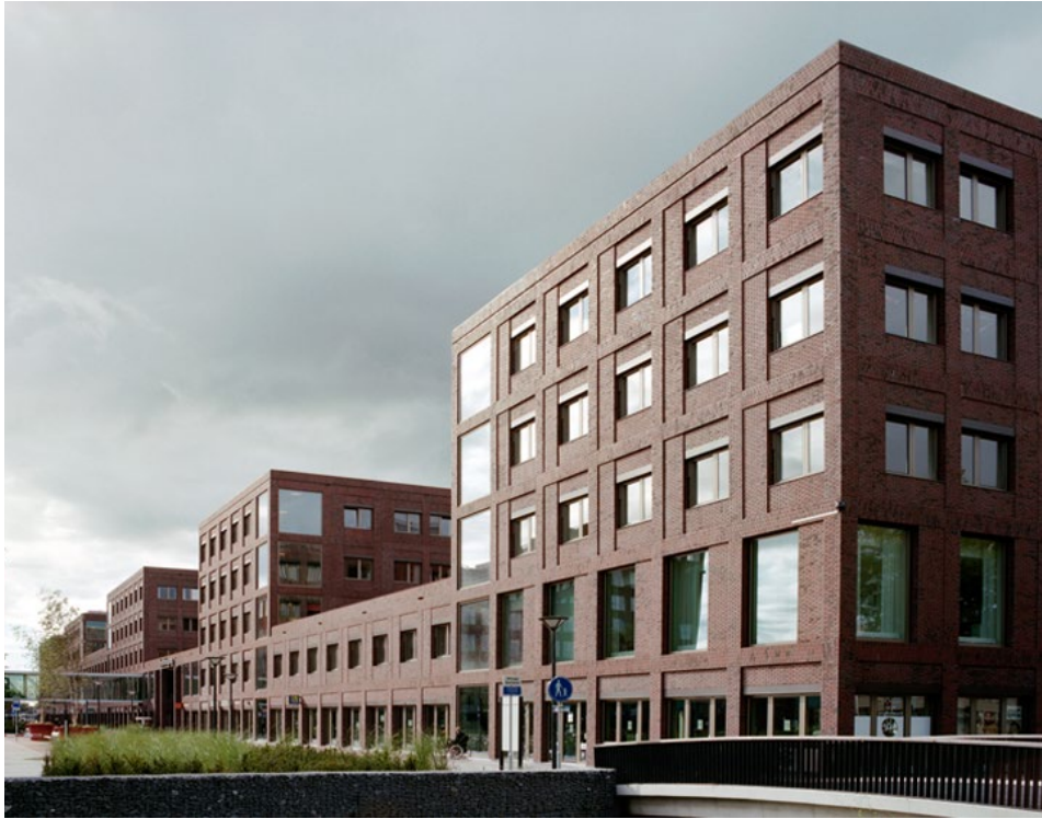
Maasstad hospital, Wiegierinck architects, 2016
