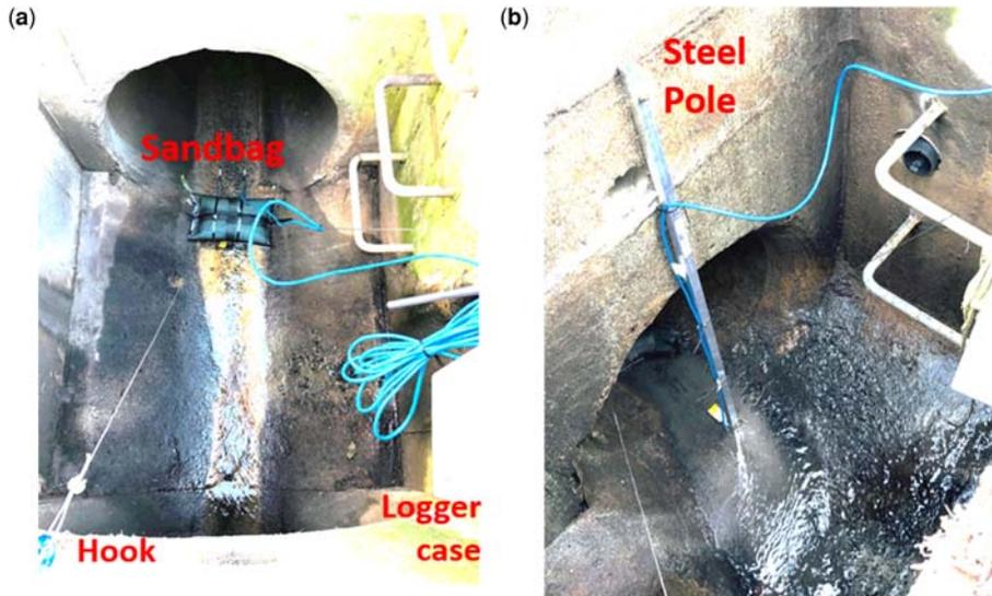
**Figure 11.17** Typical installation methods of NextGen Urban Water Monitoring sensors in drainage network – attaching to a sandbag (a), fixing a pole with anchors and connecting the sensor to the bottom of the pole (b). Source: EPHM Lab and BoSL.
