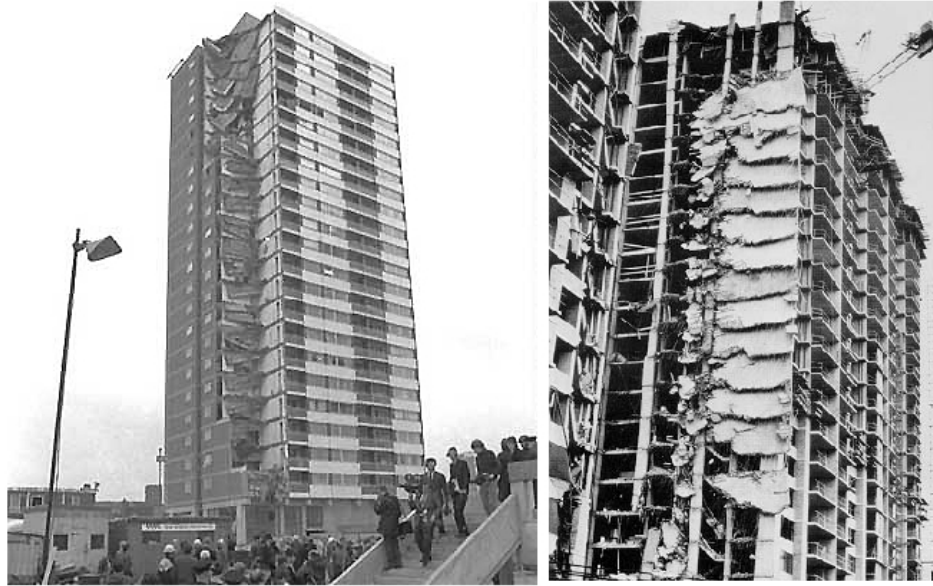
Figure 2.2: Two similar cases of progressive collapse: Ronan Point (left) and Skyline Plaza (right).
