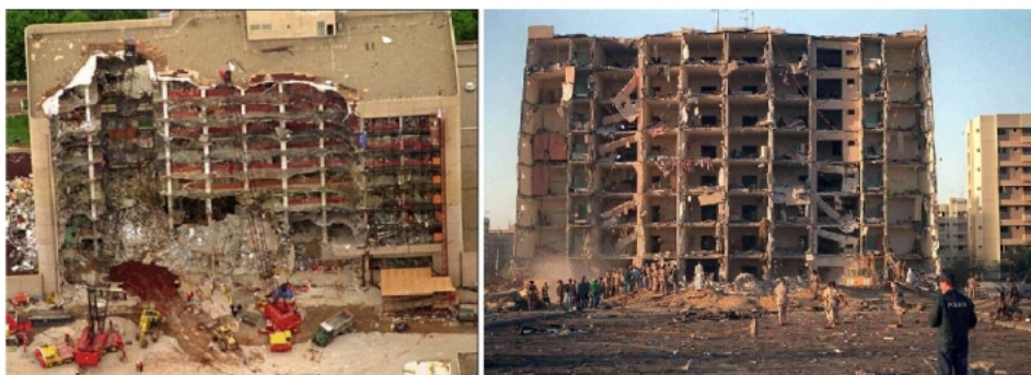
Figure 2.3: Damage to the Alfred P. Murrah building in Oklahoma (left) and the Khobar Towers (right).
