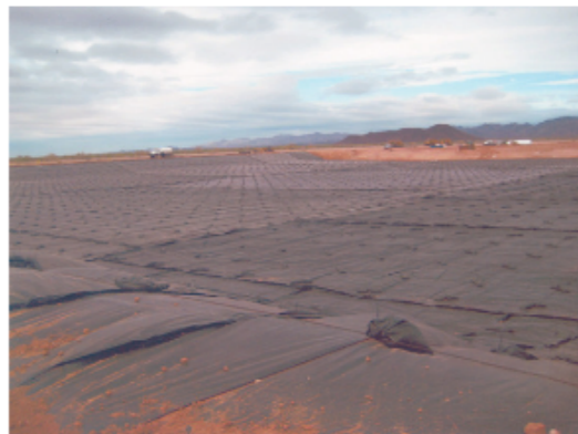
Mesquite Regional Landfill under construction, El Centro, California, 2008.
