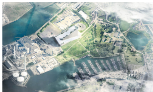
BIG, Amager Resource Center, Copenhagen, Denmark, under construction. The facility utilizes flue gas cleaning, a highly efficient technology
