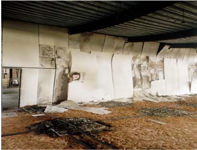
Figure 28 Instability failure of a compartment wall due to the deflection of the floor (56)
