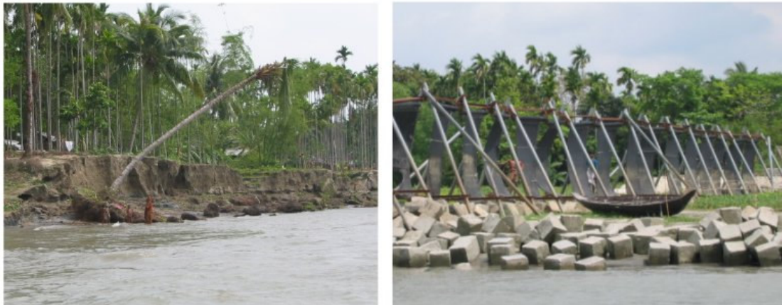
Figure 1.1: Bank erosion and bottom vane in Bangladesh
