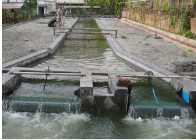
Figure 5.1: Outdoor facility BUET, Bangladesh
