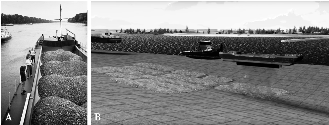
Figure 1.4: Sediment nourishments with barges. Image courtesy: A. Kondolf (1997) (photograph taken below Iffezheim weir) B. Rijkswaterstaat (screenshot from animation).
