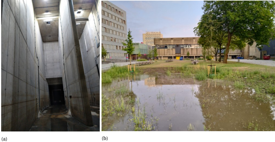
Figure 1.1: Examples of UDS improvement for CSO reduction with (a) an example of a stormwater tank, taken from the Graz sewer system and (b) a filled WADI at the Delft University of Technology Campus.
