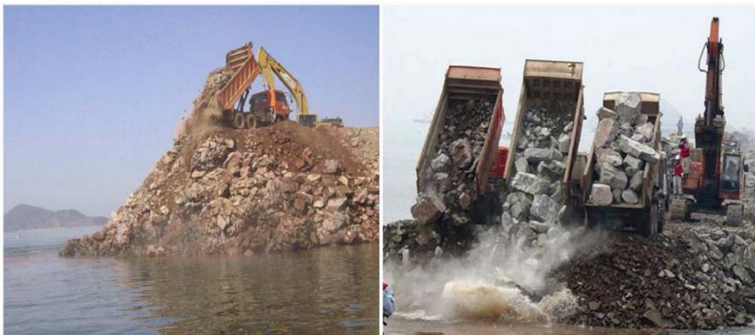
*Figure 2-12 Dumping of material over dam head*
