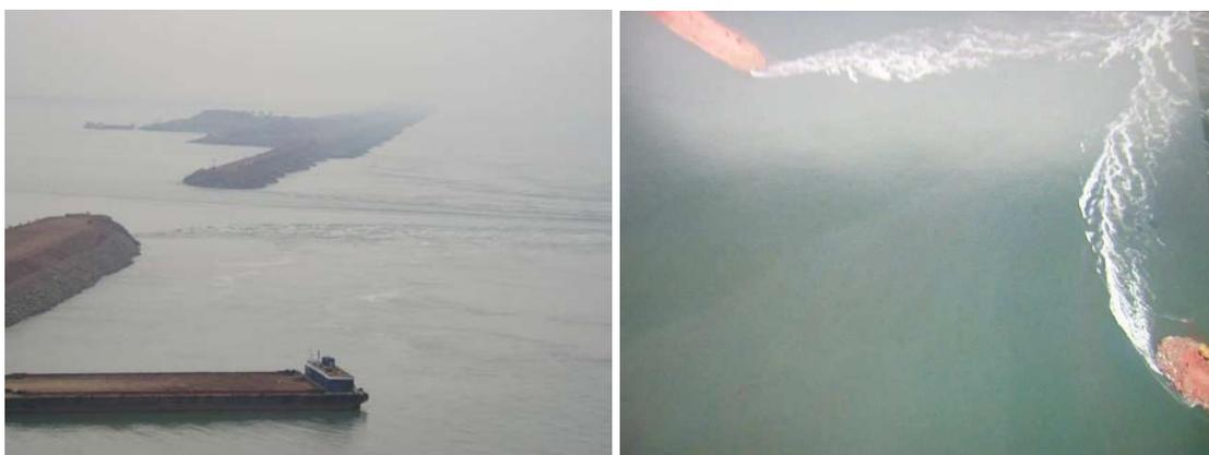
Figure 2-3 Flow pattern through closure gaps
