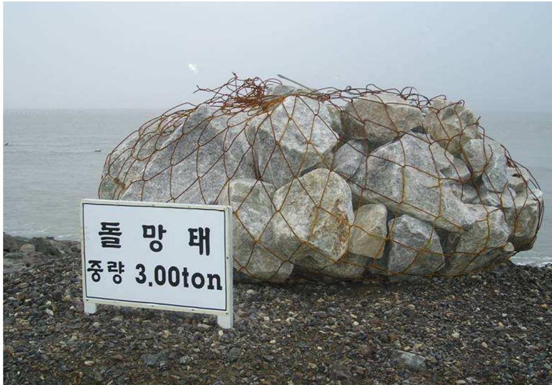
Figure 2-13 Gabion of 3 ton
