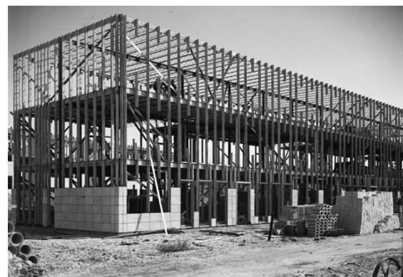
Figure 8. Scene of the NeMaVo Airey system building during the construction. (beeldbank.amsterdam.nl)
