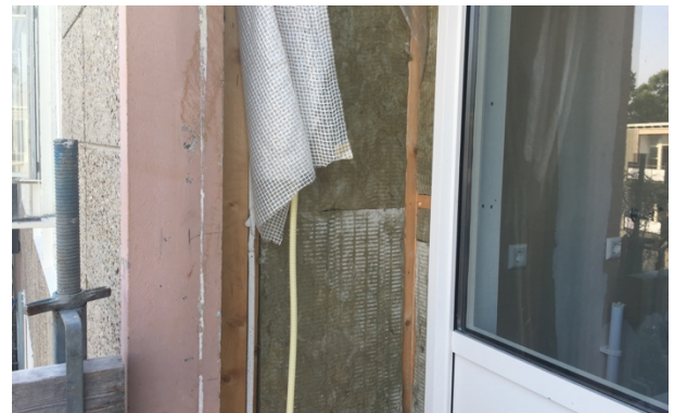
Figure 19. filling the cavity with the insulation in the current renovation project (one image)
