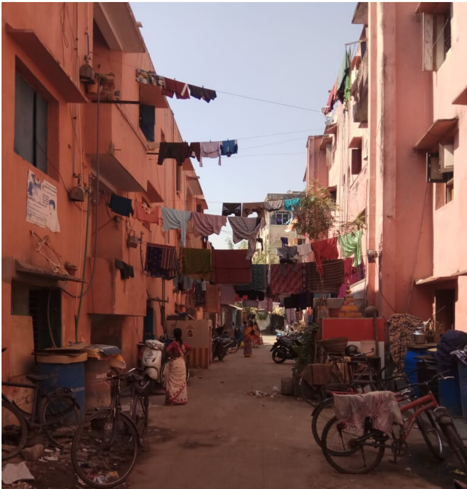
Figure 30. Existing building (Tamil Nadu Slum Clearance Board Housing) along the Mambalam canal (Pictures taken by the author, March 2019)
