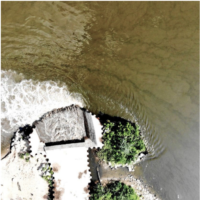
Fig. 22. Sewage leaking the Vistula River after a failure of the wastewater treatment in Warsaw | September 2019 Source: photograph taken by Maciej Jazwiecki | Agencja Gazeta | polityka.pl
