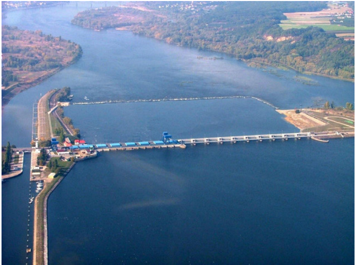
Fig. 30. Wloclawek dam, view from the side of the upper reservoir Source: Szymkiewicz (2017)
