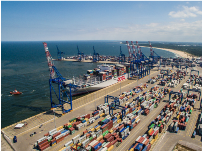
Fig. 28. Deep-water Container Terminal in Gdansk Source: gospodarkapolska.pl
