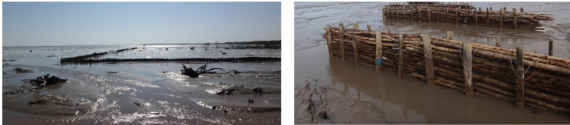
Figure 1.6: Picture showing the rows of permeable dams that make up the STUs constructed at Weg naar Zee
