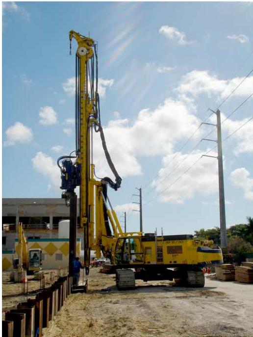
Figure 39-2 Driving a sheet pile
