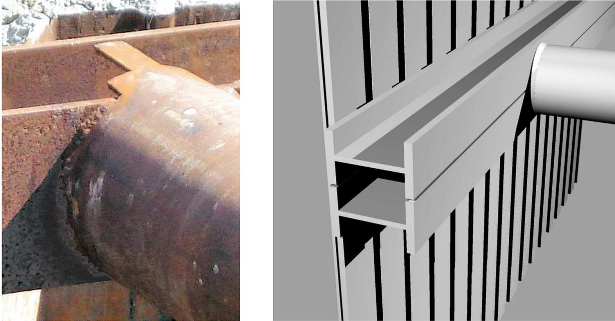
Figure 36-3 Welded connection of pipe strut and waling. The picture on the left (cofferdam near Sebastiaansbrug in Delft, 2007) shows a wale consisting of single H-profile, whereas the drawing on the right depicts the more common case of a double profile.
