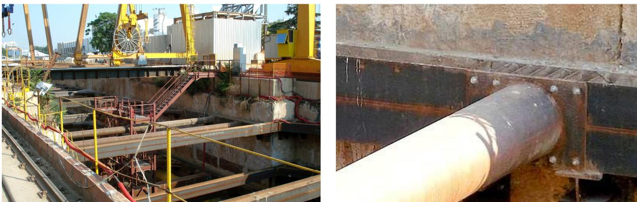
Figure 36-9 Cofferdam for the construction of the metro line in Thessaloniki, with bolt connections struts-wales (August 2009)
