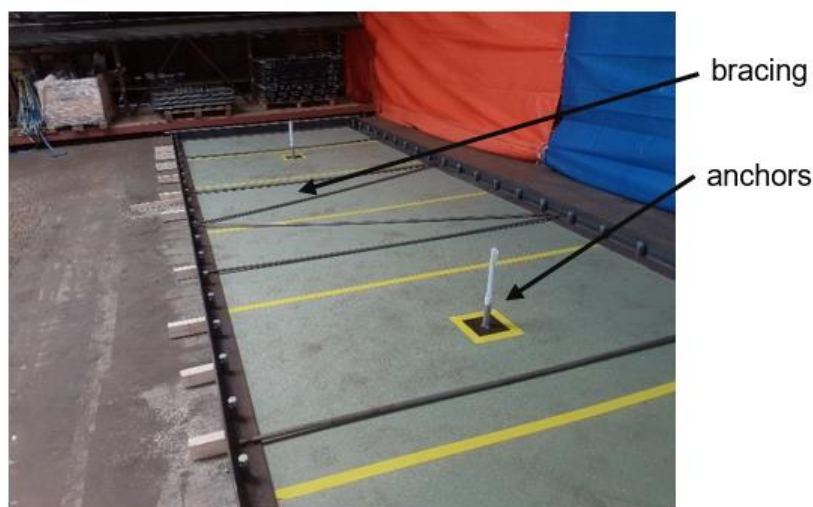
Figure 3.8 Formwork and connector installation
