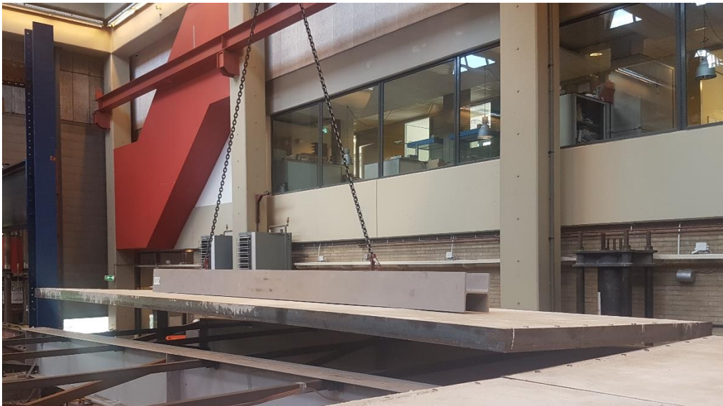
Figure 3.12 Installation of deck
