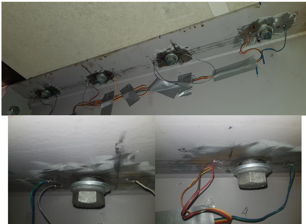
Figure 3.20 Installation of the resin injection bolts in oversized holes (12mm clearance)
