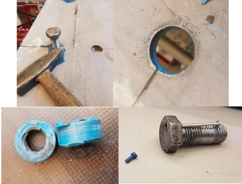
Figure 3.54 Removing resin plug and cleaned injection bolt
