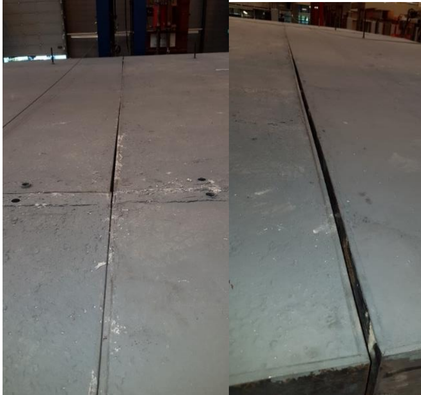
Figure 3.44 Picture from mid-span to supports and from supports to mid-span
