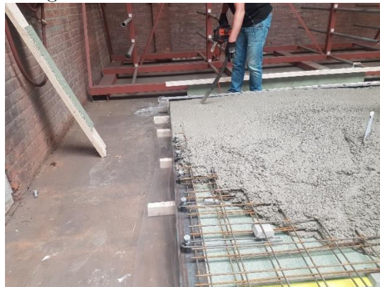
Figure 3.11 Concrete pouring and vibrating
