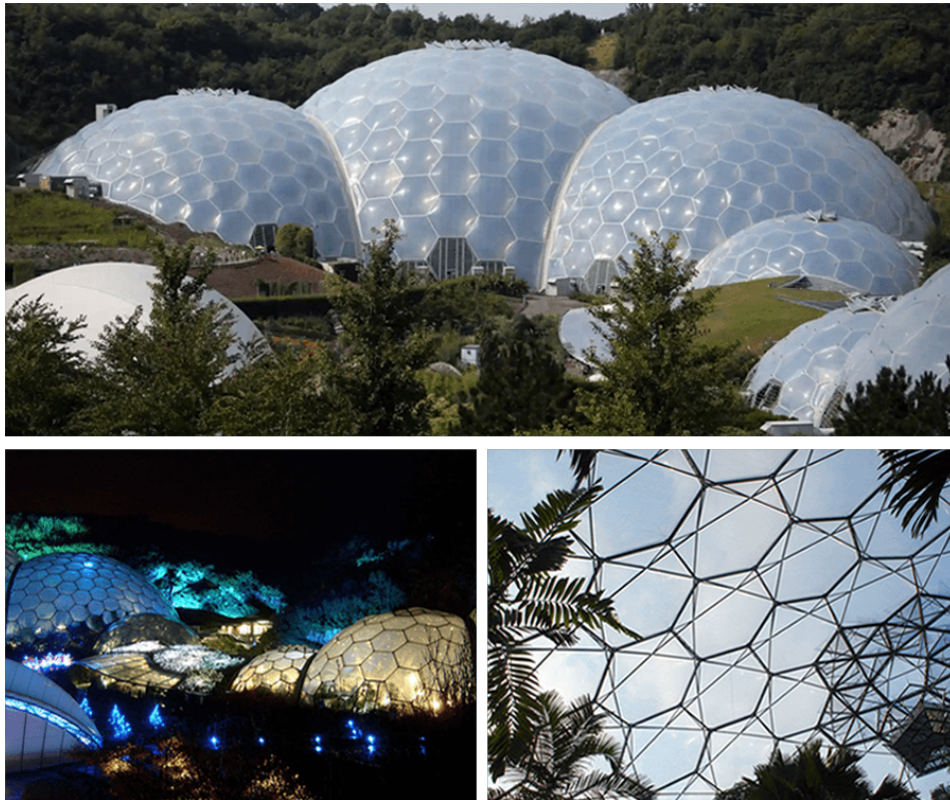
Figure 2.13: ETFE foil cushions-The Eden Project, Cornwall. [14]
