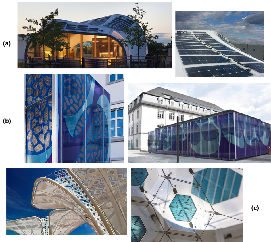
Figure 2.49: (a) Techstyle Haus - Mechanical integration [52], (b) Merck KGaA building - Lamination [57][27], (c) Germaon pavilion at Milan EXPO 2015 - Direct printing [38].
