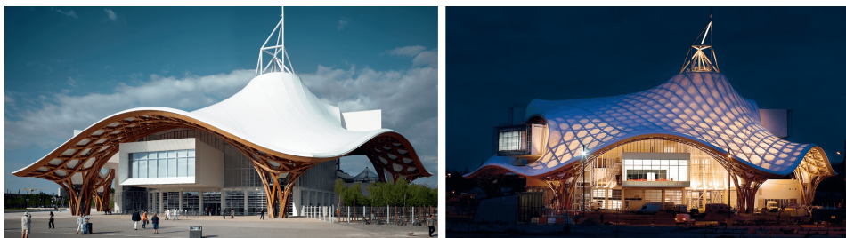
Figure 2.10: PTFE/Glassfiber fabric-Pompidou Center, Metz. [41]
