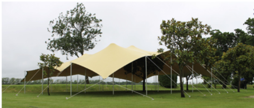
Figure 2.18: Tent structure from coated knit fabric. [20]
