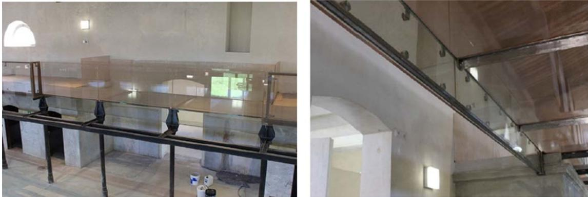
Figure 2-25 reinforced laminated glass beam of the glass footbridge (Mamone, Masiello, Lani. 2016)
