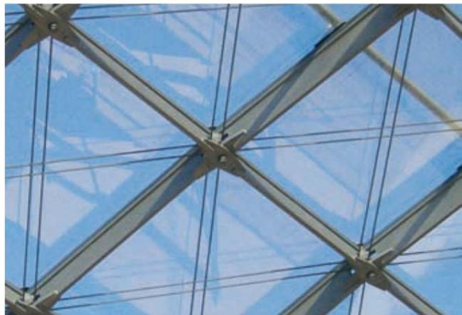
Figure 2-5 Section and facade using clamped connection (Structural use of glass in building)
