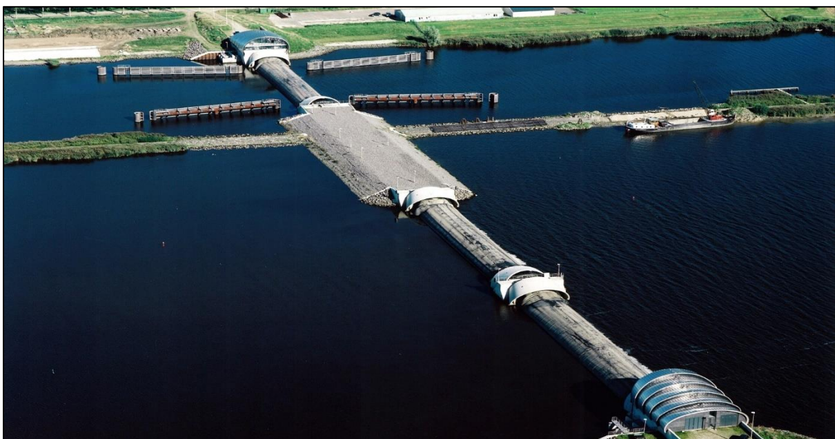
Figure 3 Ramspol Barrier during closing state [9]
