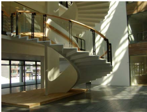
Fig. 2. Staircase of UHPFRC in Denmark (Courtesy B. Aarup [2]).
