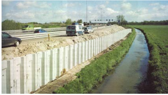
Fig. 10. Earth retaining wall of concrete sheet piles
