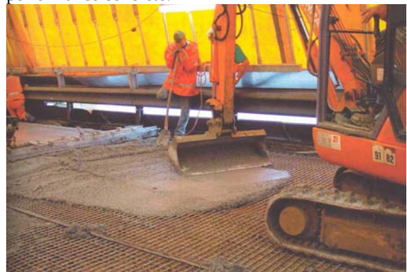
Fig. 12. Spreading the concrete at the site
