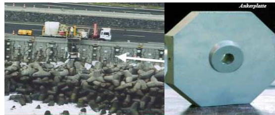
Fig. 6. Application of HPFRC for prestressing anchors in a coastal area (Ile de la Reunion, [7])
