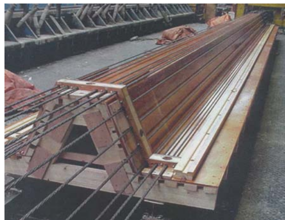
Fig. 9. Formwork for a high performance fiber reinforced sheet pile, Spanbeton, The Netherlands
