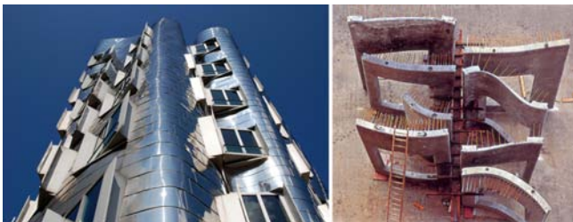
Figure 1. Der Neue Zollhof, Düsseldorf: final result and the underlying pre-cast elements
