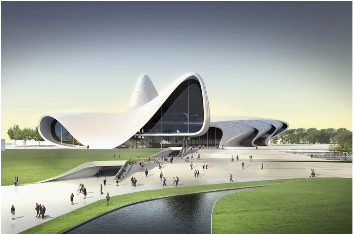
Figure 1. Exterior View of Main Entrance
