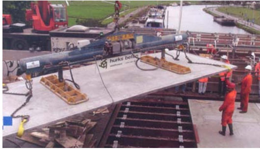
Fig. 13. Assembly of precast bridge deck panels in reinforced ultra high strength fiber reinforced concrete (Kaag Bridges, The Netherlands, 2003)
