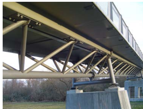
Fig. 3. Gärtnerplatzbridge in Kassel, Germany (2007), consisting of a high performance deck glued to a 3-D steel truss
