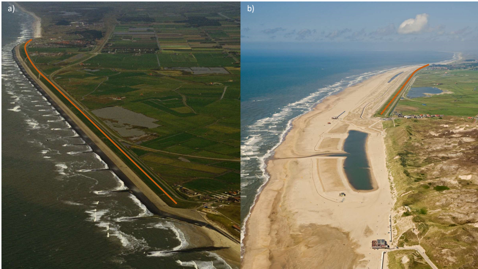
Figure 2.1.: a) Hondsbossche sea dike before placement of the nourishment (courtesy of Rijkswaterstaat, https://beeldbank.rws.nl/ , accessed on 6 September 2021) and b) the Hondsbossche Dunes Nourishment just after placement in April 2015 (courtesy of Annemerscombinatie Zwakke Schakel–Van Oord-Boskalis). The orange line marks the crest of the original sea dike.
