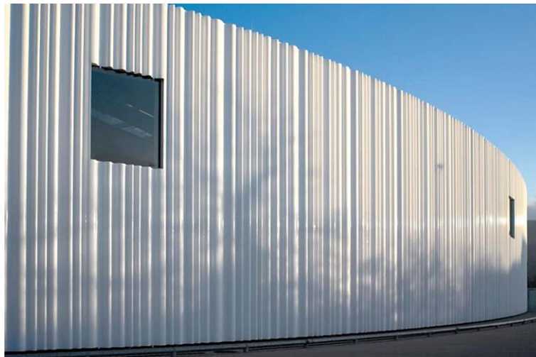
Fig. 4. Completed façade section (Image: Michel).
