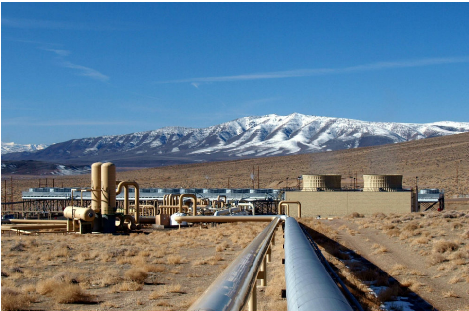
Figure 1.2: Geothermal ORC power plant of 22 MW installed by Ormat in the Churchill County of Nevada. (22)
