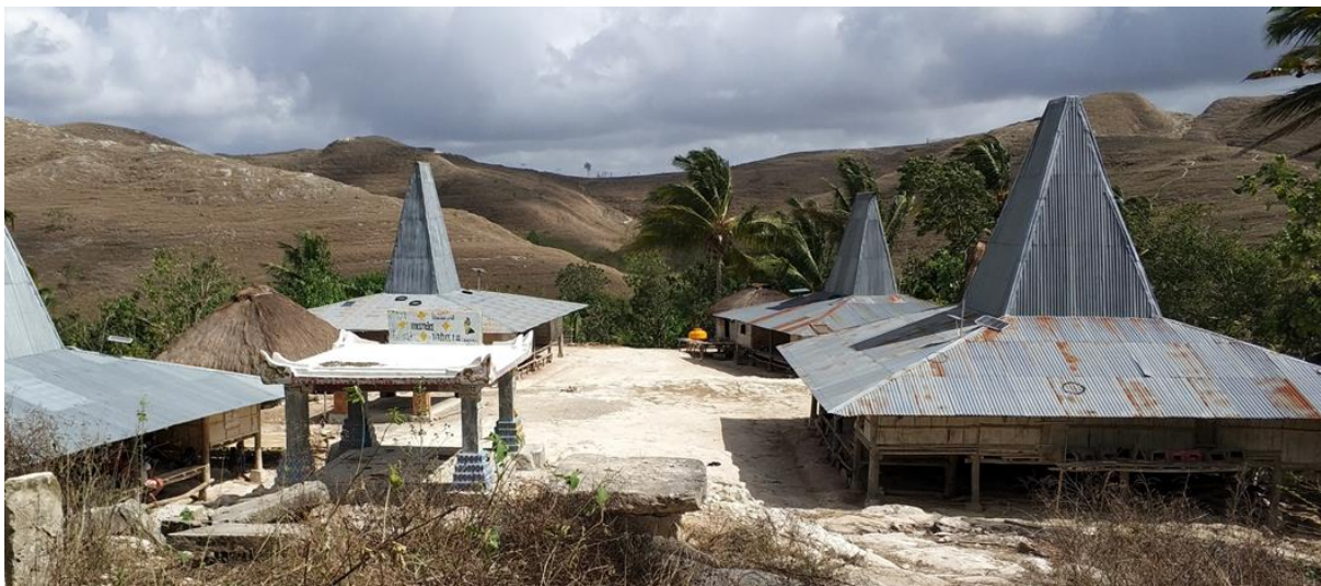
Figure 4. The traditional Sumbanese, stilt, house in one sub-village in East Sumba and the surrounding environment. Picture was taken by the first author.
