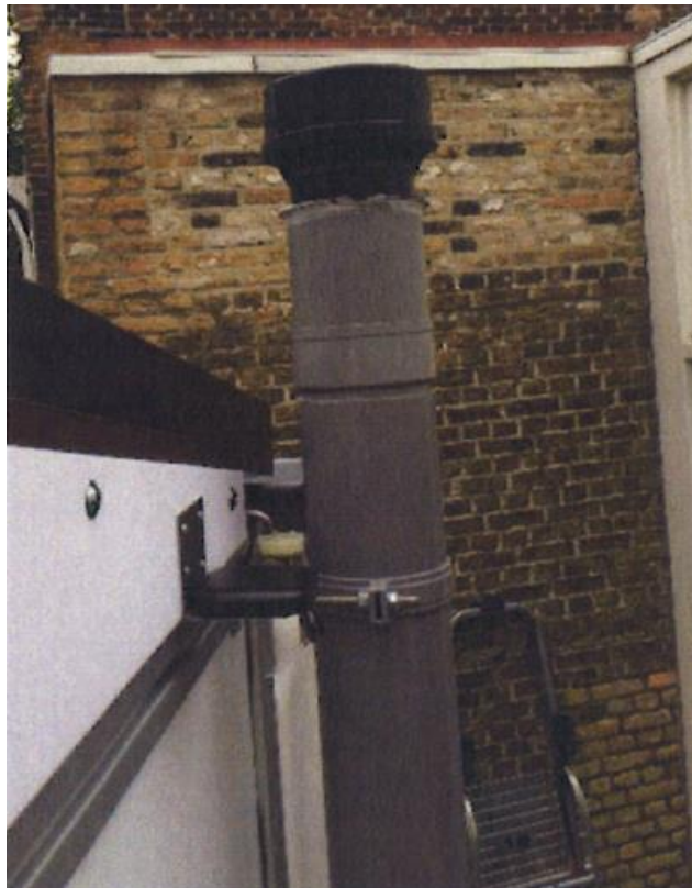
Figure 3-21 Granular activated filter for odour control in experimental eSOS Smart Toilet (Photo: J. Ćurko)
