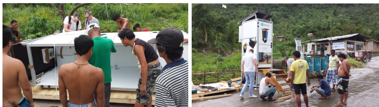
Figure 3-37 Assembling the toilet on-site with the help of local community (Photos: F. Zakaria)
