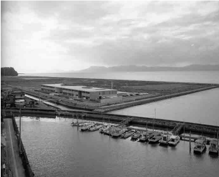
Fig 28. The building fabric perfectly fits within the horizon of the artificial landscape.
