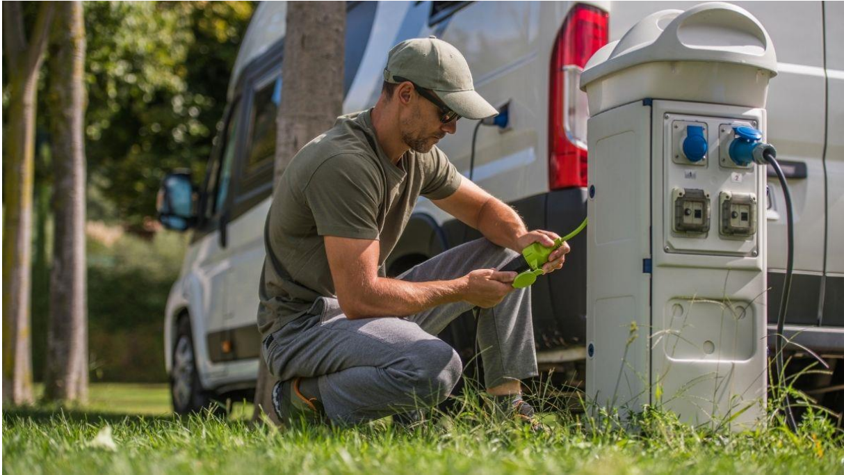
Figure K.18 Connecting to the campground power grid
