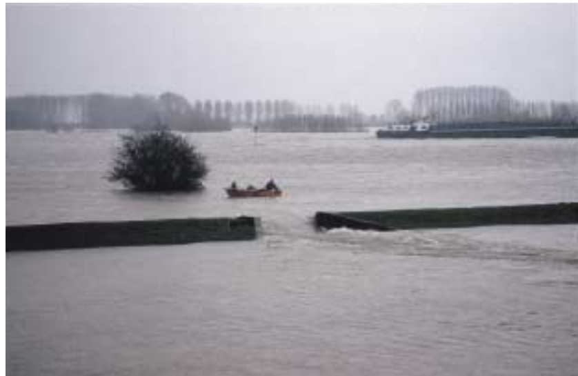
..... Figure 7.2 Minor embankment with inlet during flood (photo: Henk Wolters).
