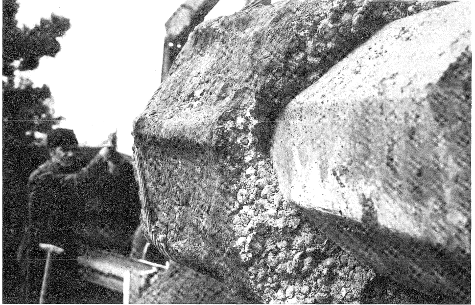
Fig. 11. Photograph of deteriorated lamp post.
