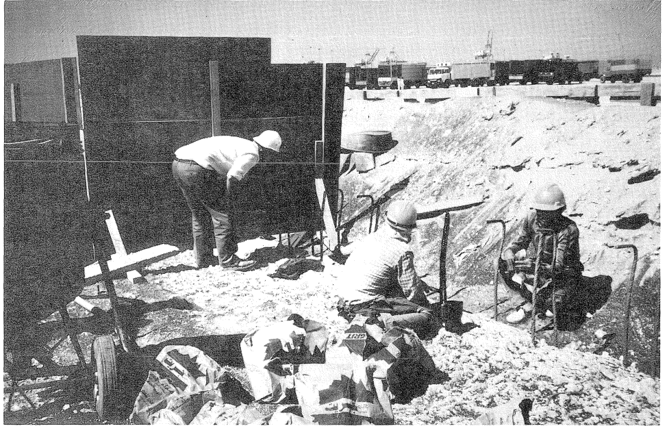
Fig. 42. Photograph of the coating operation of steel reinforcement during the repair of the Al-Shindagah Tunnel in Dubai.
