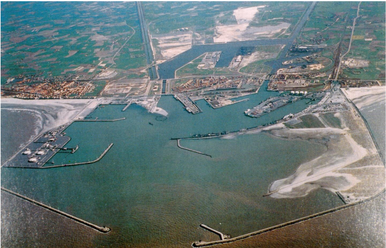
Figure 1.1: Rubble mound breakwaters at Zeebrugge, Belgium ( http://www.kennisbank-waterbouw.nl )
