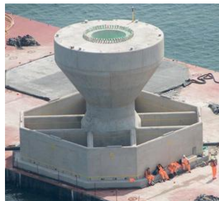
Figure 7, Standard design GBF with ice cone
