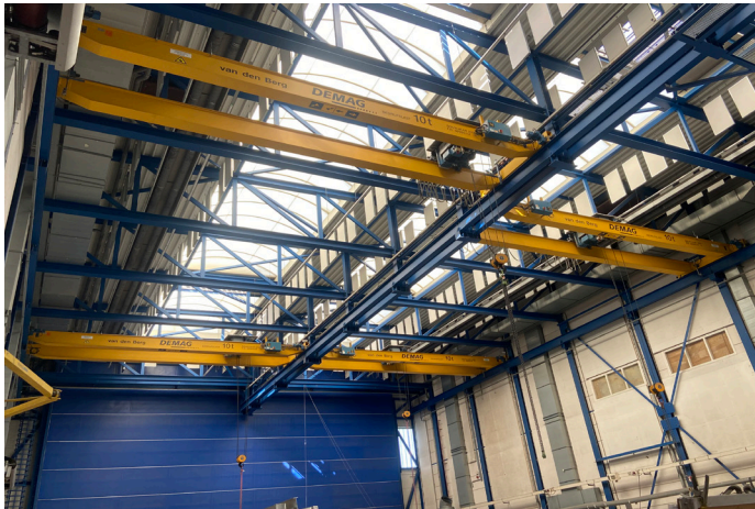
Figure 24: The overhead cranes (yellow) in hall two in Leiden.
