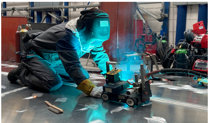
Figure 15: A welder welding the hull plates together with the buggy.
