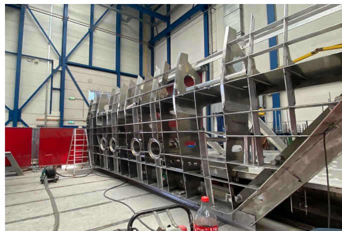
Figure 19: The structure ground loose and rotated in an upright position, supported by a T-beam, to be welded.
