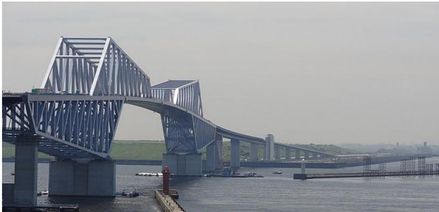
Figure 3.10 Tokyo Gate Bridge
