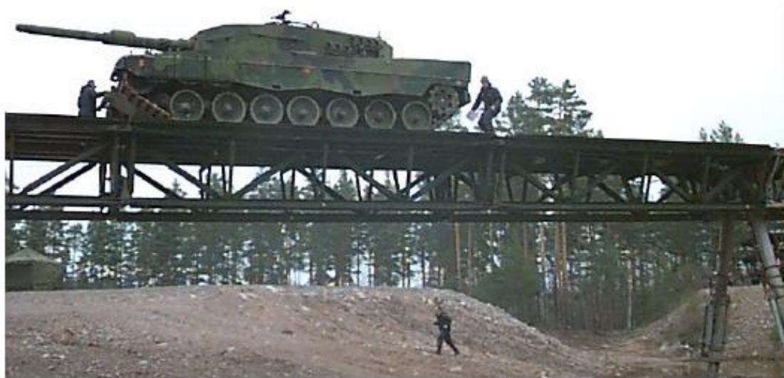
Figure 3.5 The Fast Bridge48 loaded by a tank.
