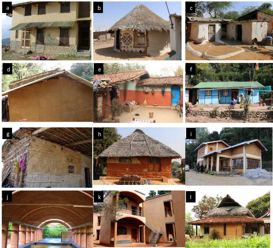
Fig. 4. (a) Adobe structure in Bir built with attention to design and engineering [owned by an organisation], (b) Traditional earthen house 'Bhunga' in Khavda, (c) Adobe house with metal roof in Kriparampura, (d) Cob house with asbestos roof in Serjtkhel, Khunti, (e) Cob house with country fired curved tile in Tangerpalli, Sundargarh, (f) 'Ikara' house with metal roof in Namchi, (g) Under construction house in Delhi [split bamboo and grass visible on walls], (h) Earth bag house with thatch roof in Tiruvannamalai, (i) CSEB house in Namchi, (j) CSEB arch structure near Pondicherry [9.5 m span and 42 m length is 10 cm thick], (k) Poured earth houses near Pondicherry and (l) rammed earth wall with country fired brick tiles and thatch roof in Tiruvannamalai.
