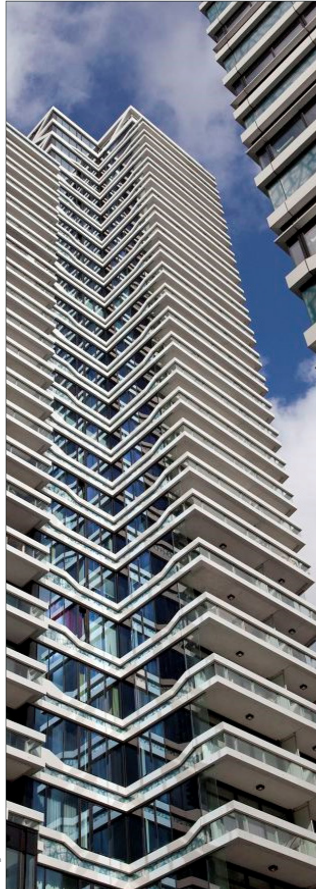
Figure 24a. New Babylon towers by J. Brobbel in De Architect, 2013
