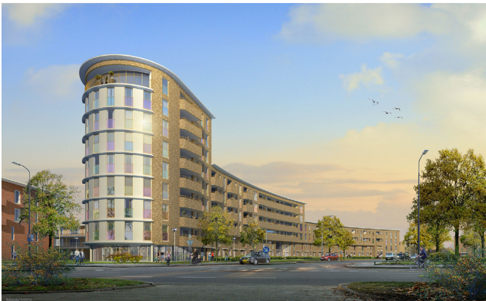
Figure 6-14: North West side of De Groene Hoven when finished (source www.degroenehoven.nl , retrieved October 25, 2010)
