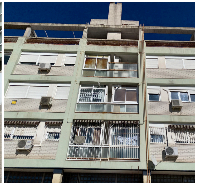
Improvised Balcony Extensions Lack Horizontal Shading
