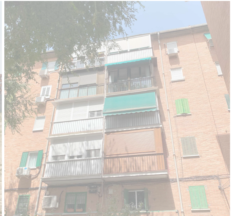
Improvised Balcony Extensions Lack Horizontal Shading
