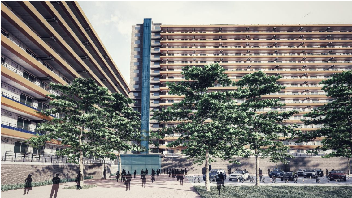
Figure 89: Entrance view of the building.
