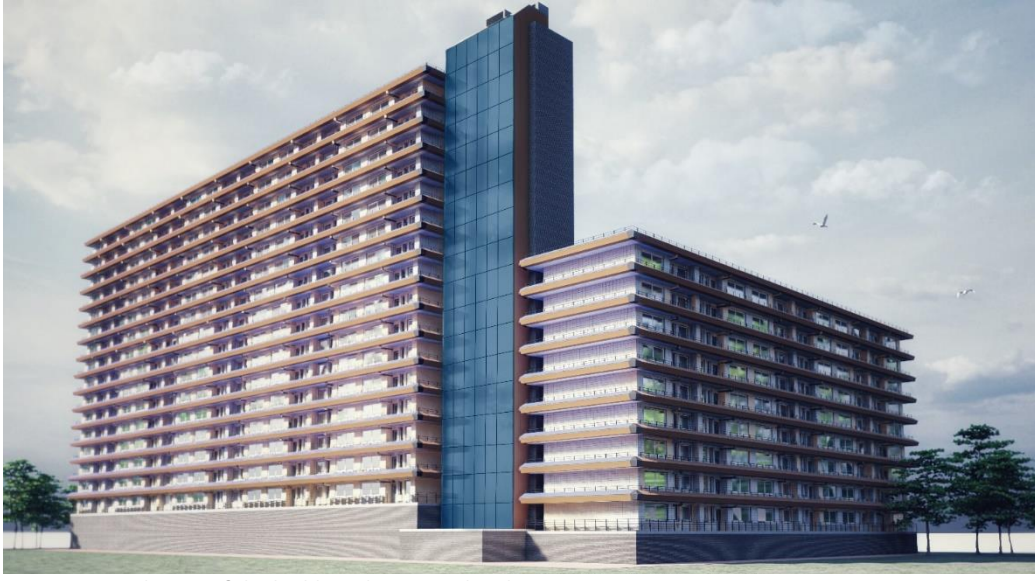
Figure 92: Back view of the building showing solar chimney.
