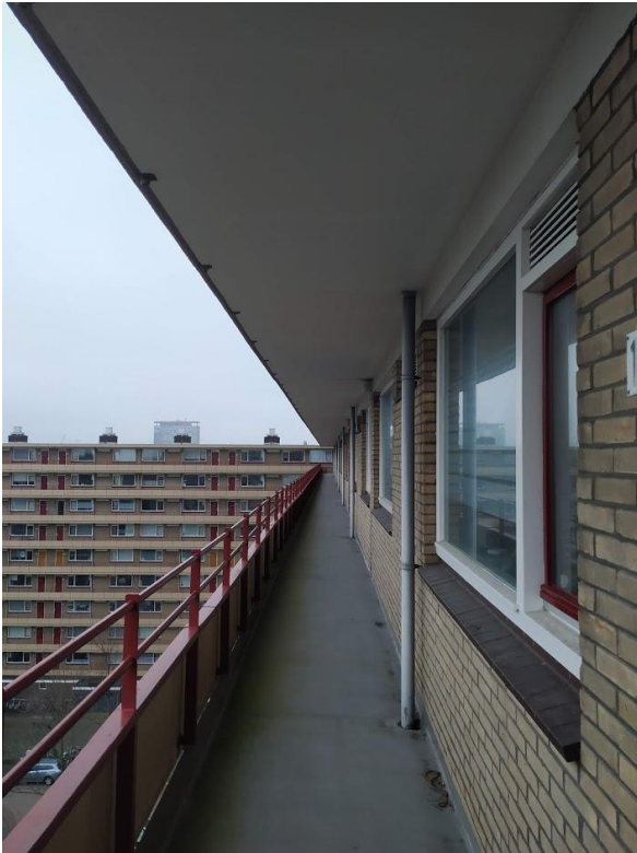
Figure 33: View through the gallery. Source: author
