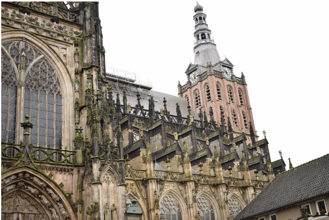
Northside of the Nave with the flying buttresses and flyer chairs and part of the north transept.
