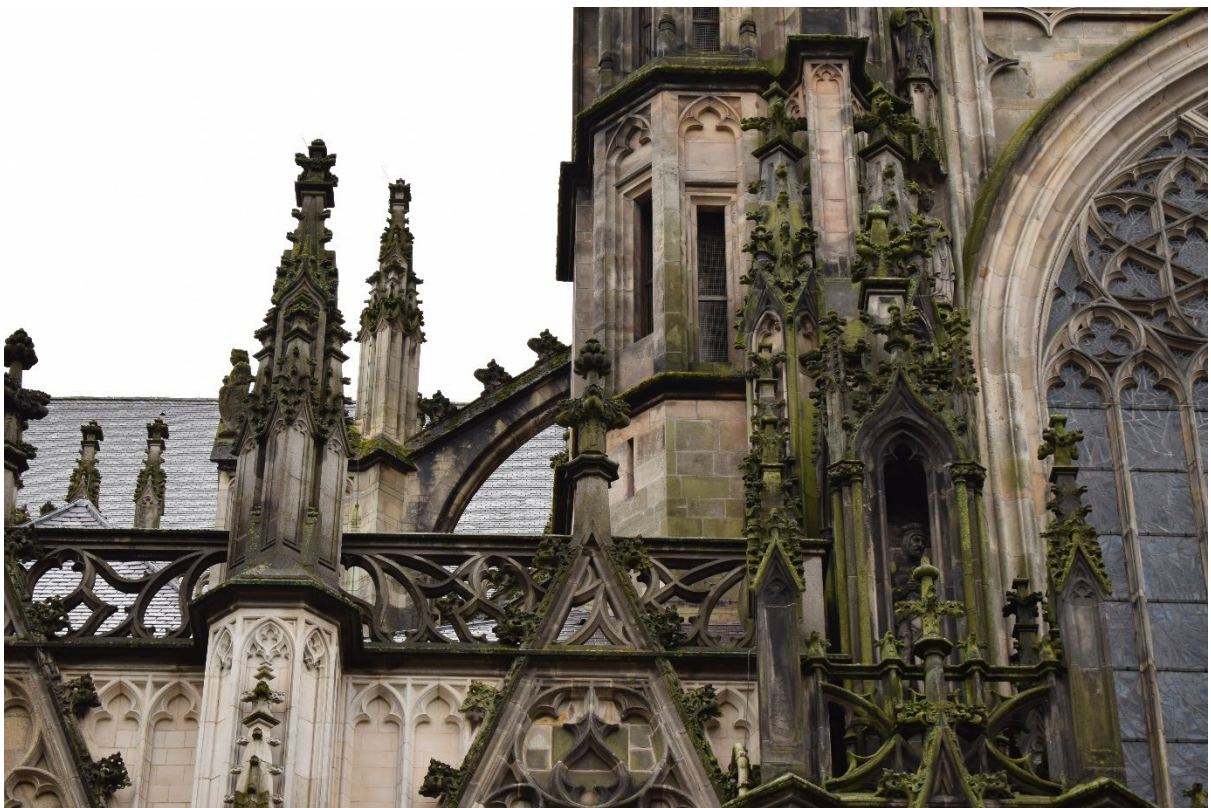
The top flying buttress on the west side of the south transept, crockets visible.
