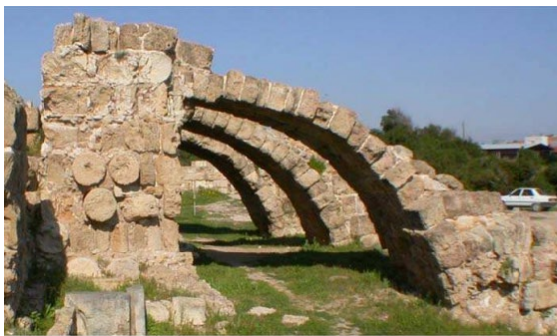
Figure 5: Early flying buttresses in Salamis-Constantia, Byzantine Cyprus 40
