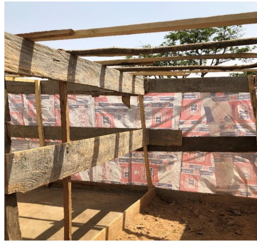
WOODEN FRAME WITH SAWN WOOD
