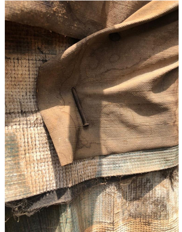
NAILS CONNECTION BENT TO SECURE PLASTIC SHEET
