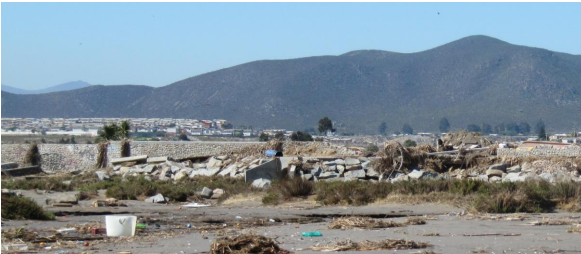
Figure III - 11: Taken right next to figure (III - 10), both the revetment and road are destroyed.
