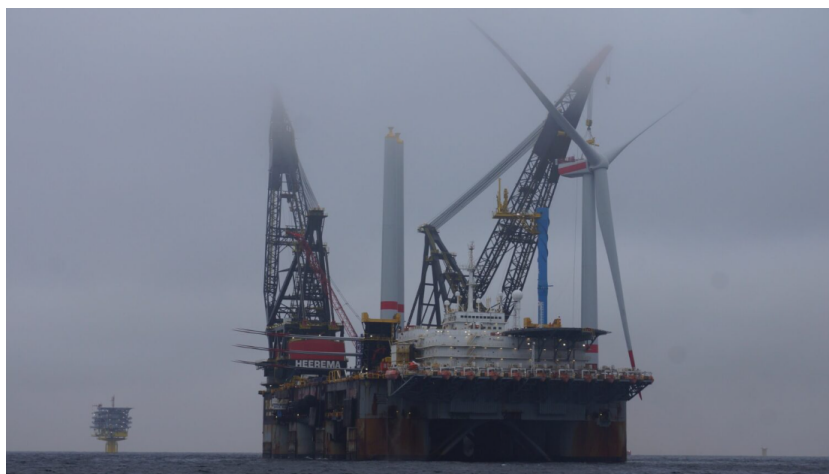
Figure 1.4: Installation of a rotor nacelle assembly by a floating semi-submersible crane vessel [11].
