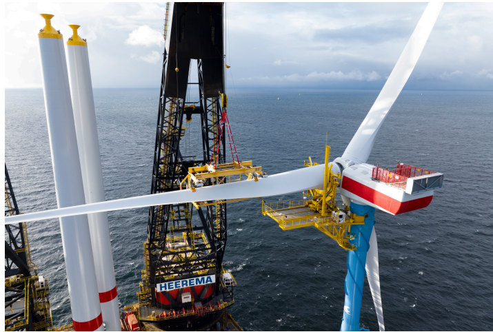
Figure 1.6: Blade installation using the GREP tool. Courtesy of Heerema Marine Contractors.
