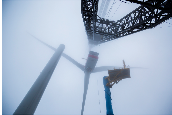
Figure 1.8: RNA installation, lifted from the installation tower on Thialf's deck to be placed on the final WTG tower. Courtesy of Heerema Marine Contractors.
