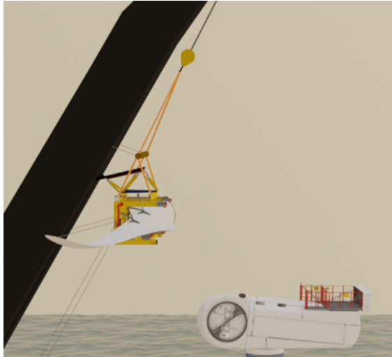
(a) Booming down and pitching the Stewart platform to keep the blade horizontal.
