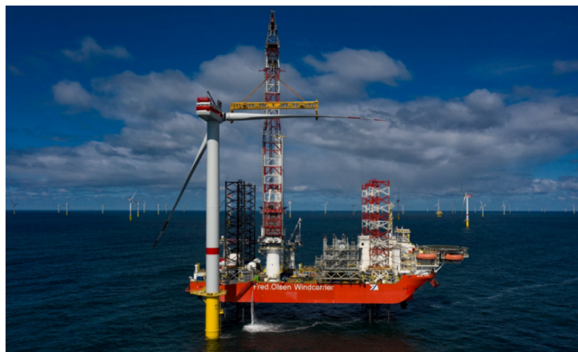
Figure 1.3: Installation of a wind turbine blade by a jack-up vessel [8].
