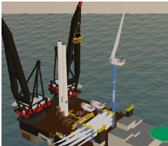
(a) Booming up, yawing the nacelle back, and rotating the hub for blade #2 installation.
