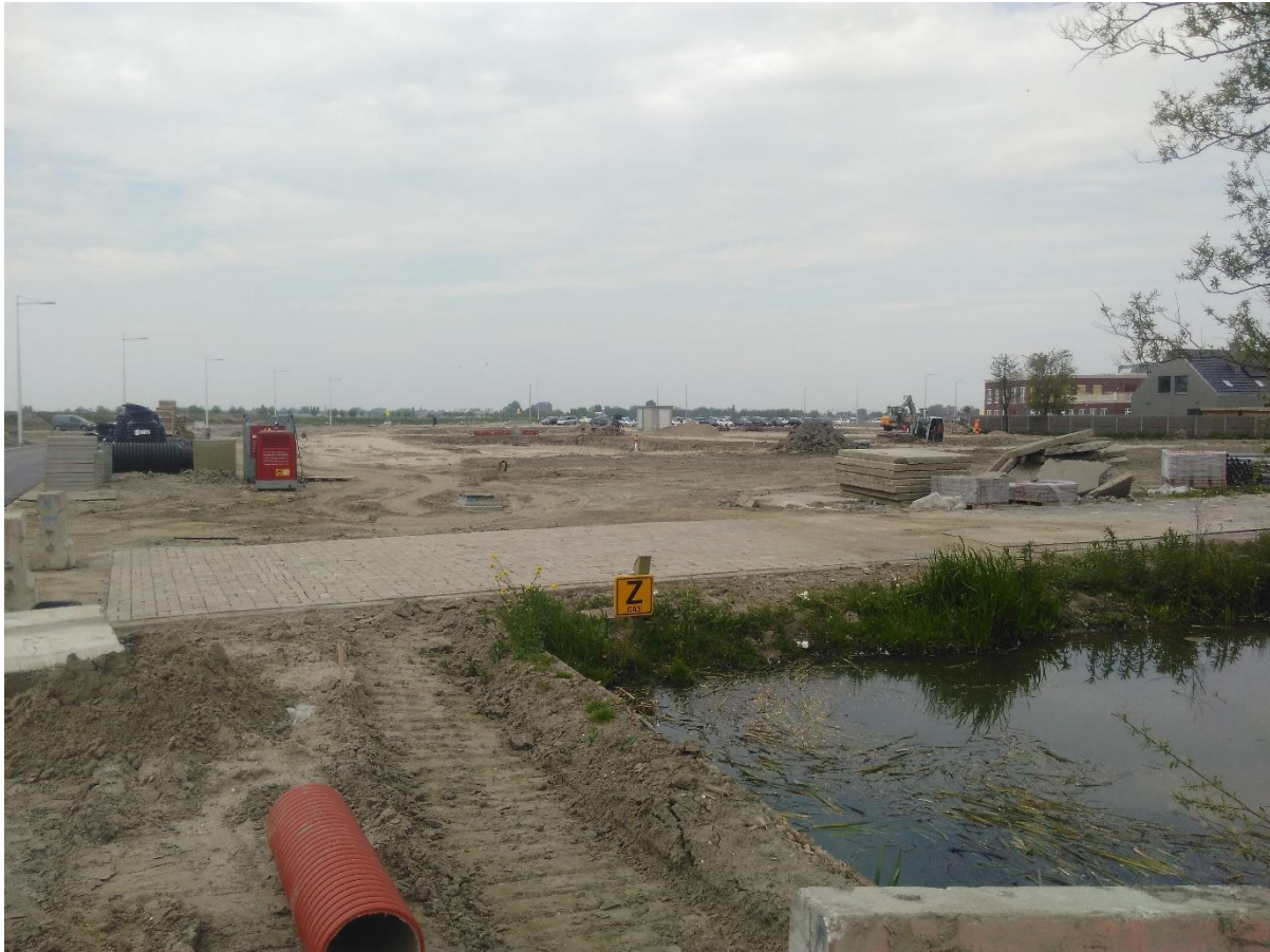
Figure 26: Impression of the construction site of Gouden Podium
