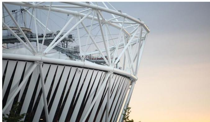
*Figure 9 – the roof trusses of the stadium made out of reused steel (International Olympic Committee, 2013)*
