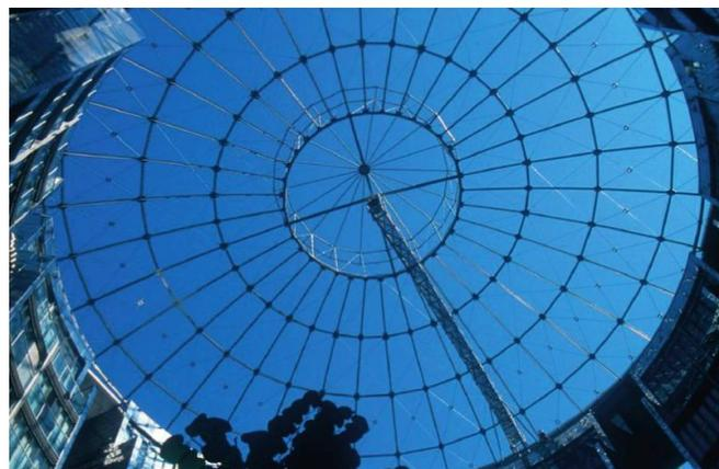
*Figure 1 - Schwedler dome on the Gasometer in Vienna circa. 1896 (Schober, 2015)*
