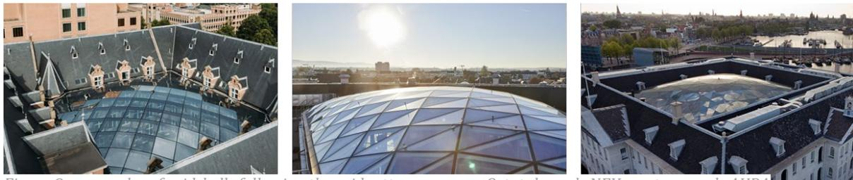
Figure 8 – examples of gridshells following the gridpattern, sources: Octatube, n.d., NEY+partners, n.d., AURA Foto Film Verlag, 2022
