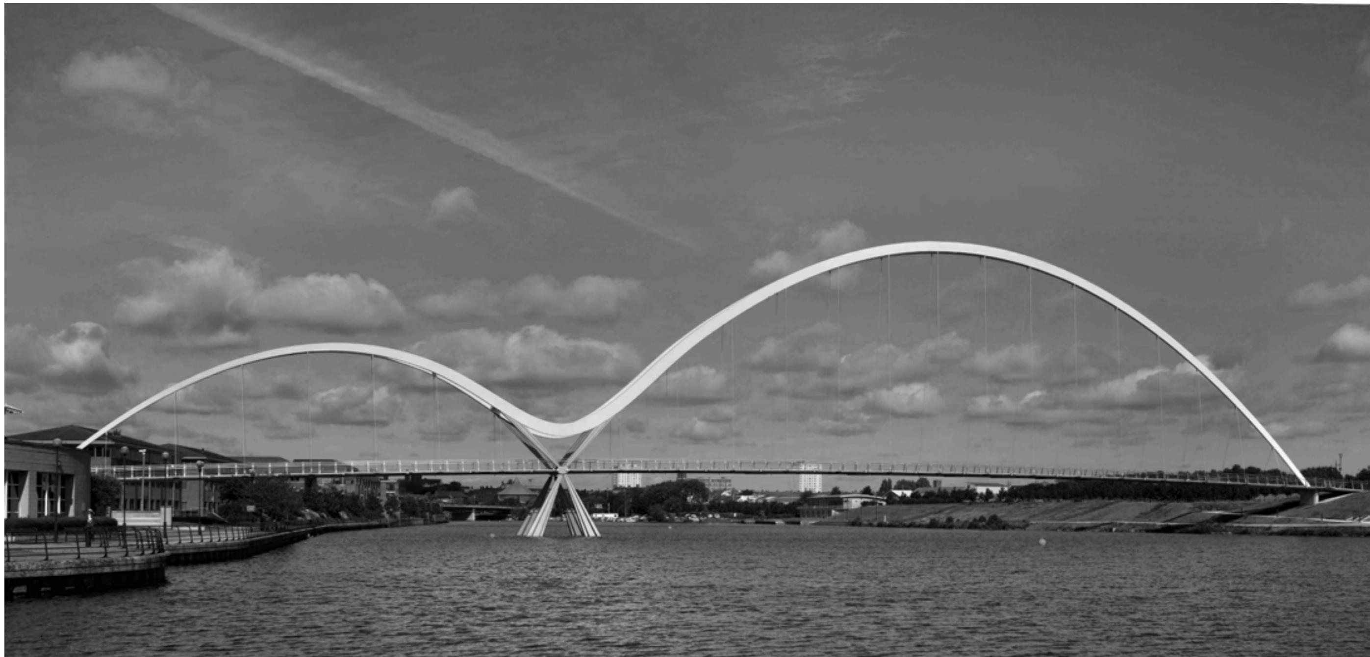
Infinity bridge door Expedition Engineering, Stockton-on-Tees
