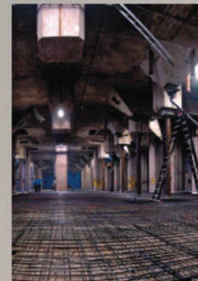
Groundfloor removing and adding columns and fortifying floor for Now & Wow 2004
