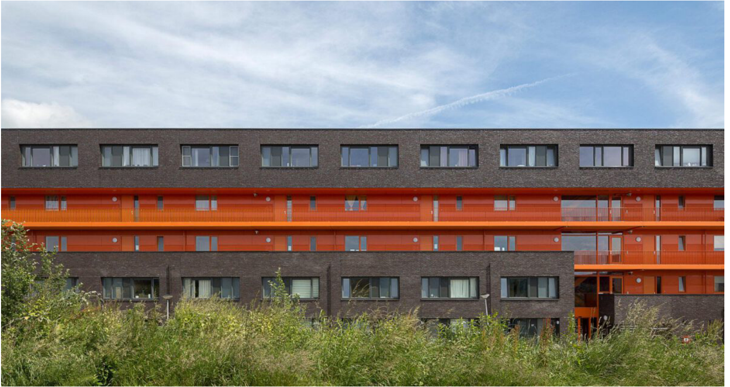
figure 7.13 West facade (Kaw Architecten 2014)
