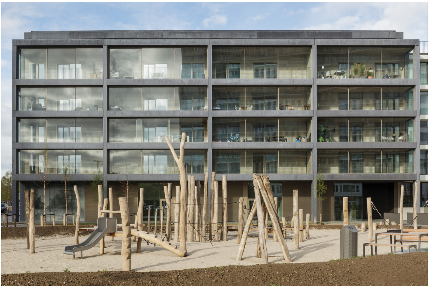
figure 7.2 Building facade (Atelier Kempe Thill, 2014)
