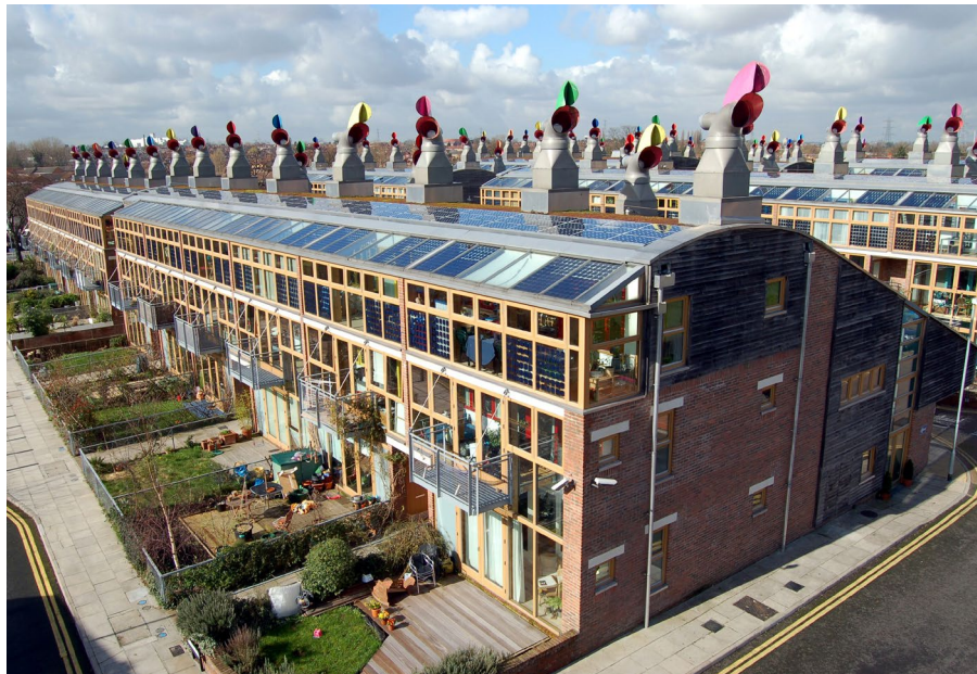
Apartment blocks, 2003. United Kingdom
