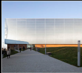
Beacon of Light Building 2018 - 11.200 m 2
